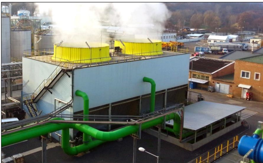
Figure 1 – The cooling tower of the Nitric Acid Plant
